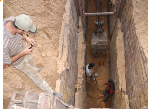
The last phase of construction works
